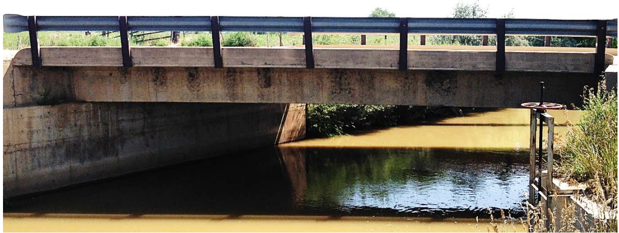
Figure 8.1 Bridge LR3-0.2-50 east elevation view
